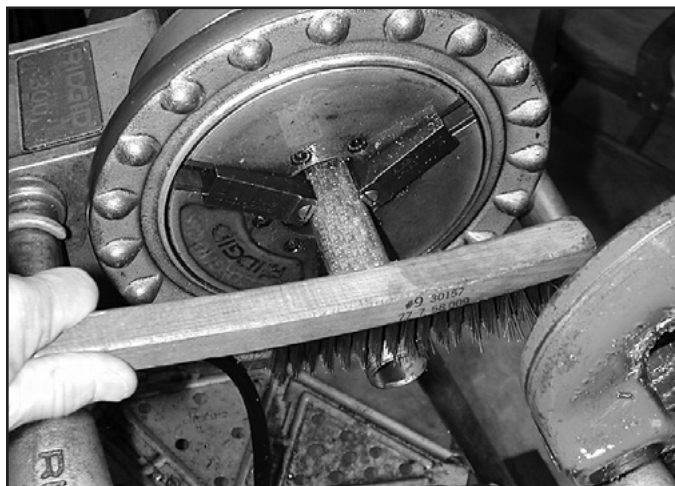
Figure 10: Wire brush the threads to remove any shavings or debris.
