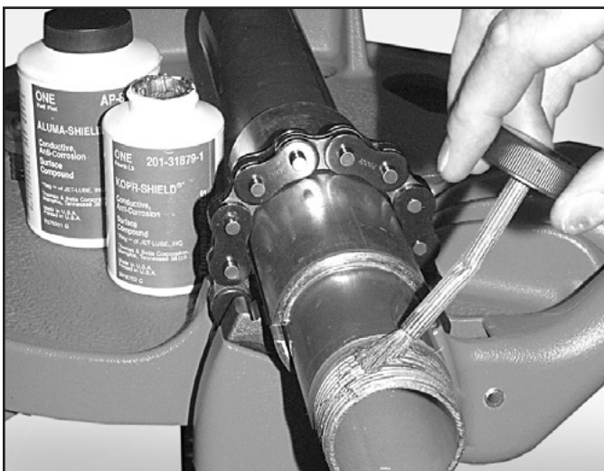
Figure 20: Application of UL listed electrically conductive corrosion protection compound on field-cut threads.
