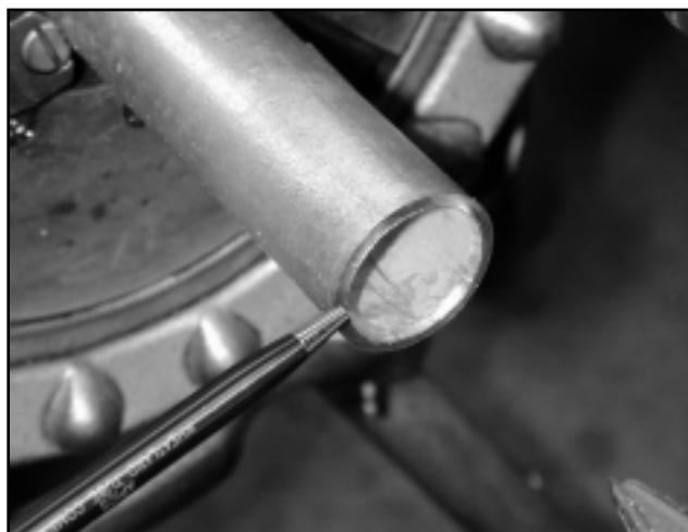
Figure 8: A minimal amount of pressure will remove the burr completely and eliminate possible flaring of the conduit end. (Courtesy of Wheatland Tube)
