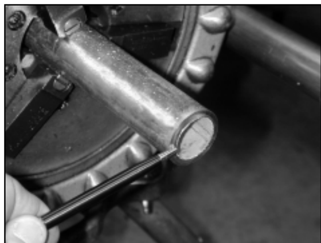
Figure 6: The roll cutter will leave a burr on the inside diameter of the conduit. The burr must be removed to ensure that the wire insulation will not be damaged during pulling. (Courtesy of Wheatland Tube)
